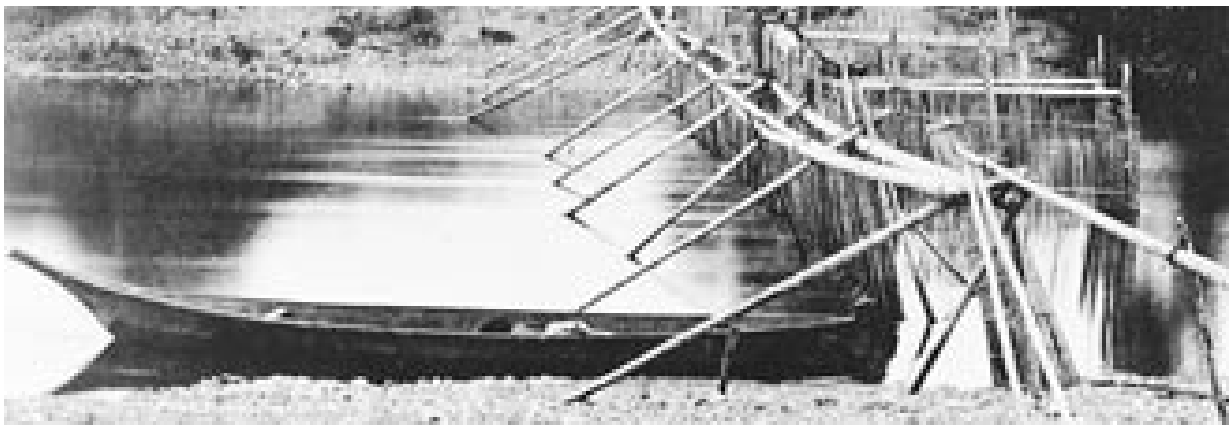
Cowichan River Salmon Weir
